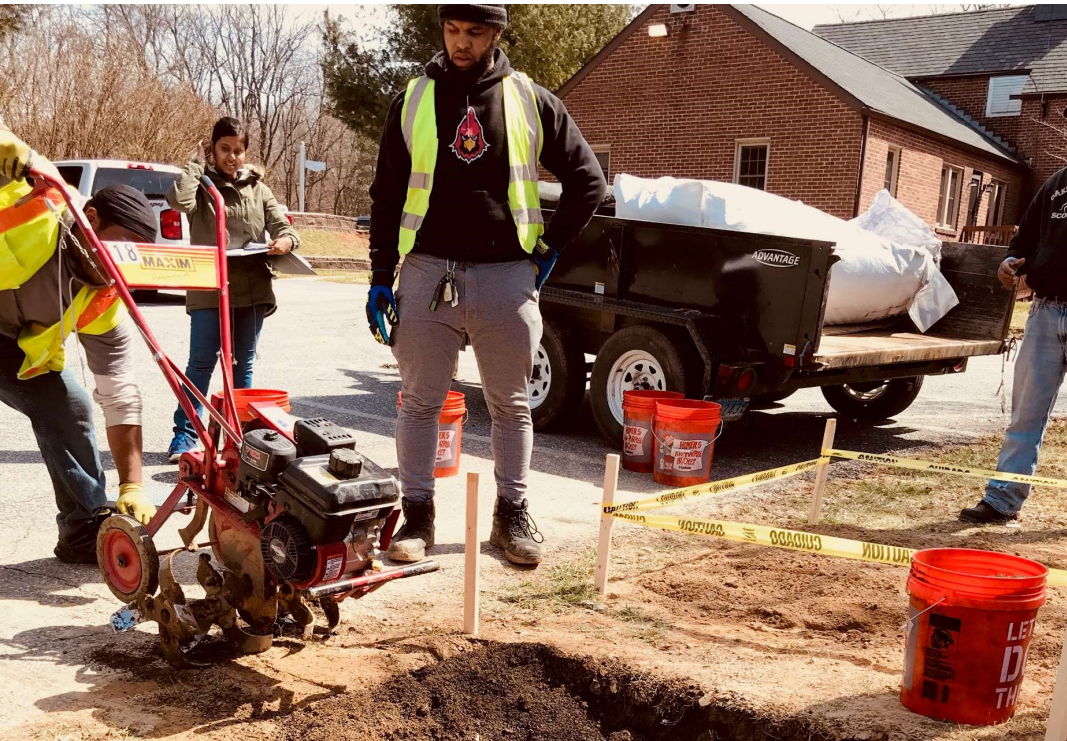
Adding and Mixing 4% by Mass Biochar
