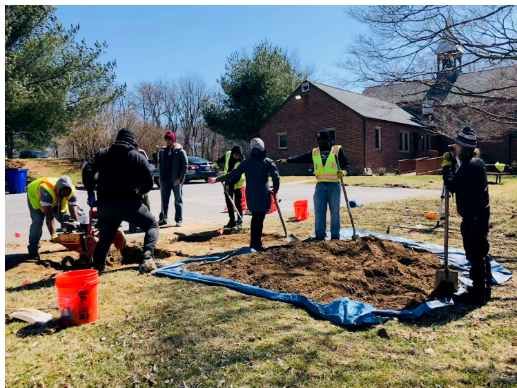
Removal of Topsoil
