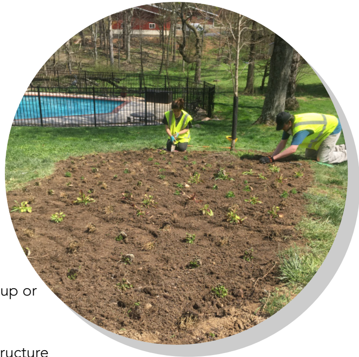
Re-grading yard away from building to landscaped area.
